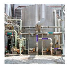
The usage of pipe markers compliant to the SANS 10140 will increase your plant safety. Those pipe markers are a combination of colours. In addition, pipe content legend and arrows can be shown. The colours to follow are indicated in the table below. The layout of the pipe itself with legend and arrows are up to the customer choice/standard.
