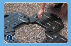
Install the "L" bolts into the slots of the rubberised plates
