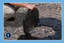
Align rubberised plates into square pattern using notches
