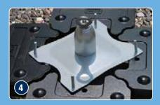
Set post and base onto the "L" bolts and plates
